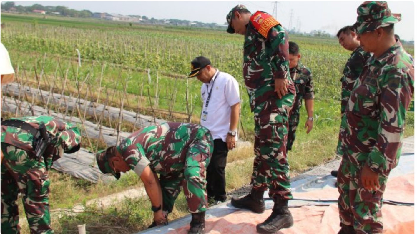
(Foto istimewa ) tim wasev cek ketebalan jalan
