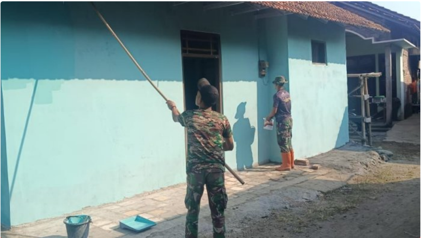
(Foto istimewa) Pengecatan RTLH TMMD 116 Kodim 0722/Kudus
